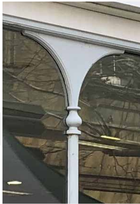
Painted timber mullion
