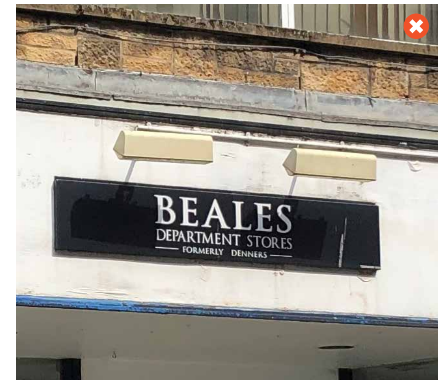
Figure 43. Lighting brackets too bulky and unattractive
