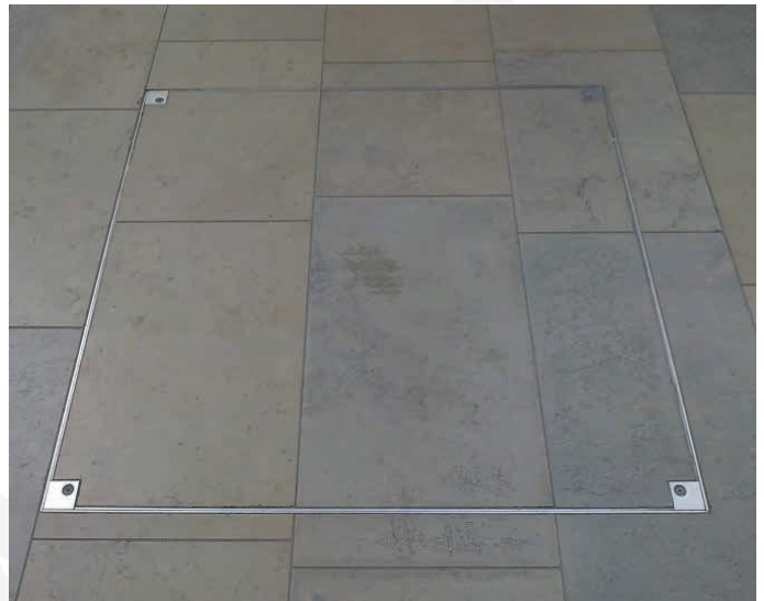
Paving infill cover
