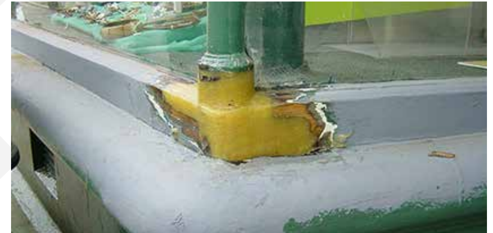
Figure 55. Resin repair to timber shopfront detail
