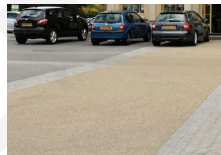
Resin-bonded Aggregate / Anti-skid Surfacing
