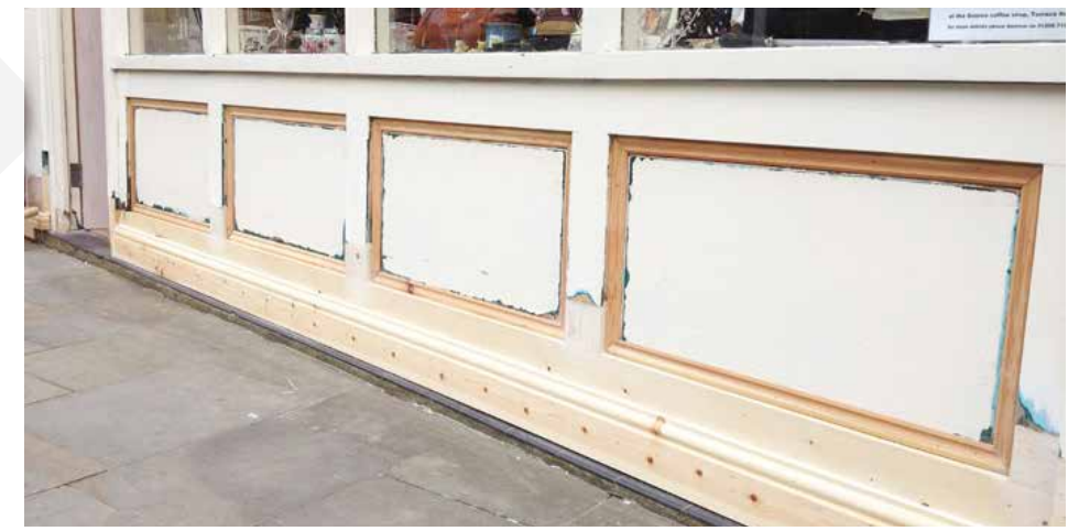
Figure 56. Timber stallriser repair
