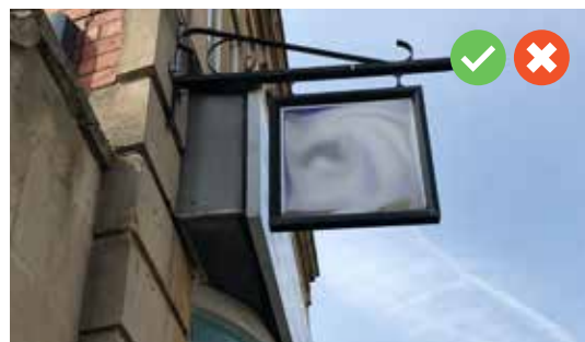
Figure 33. Hanging sign is well positioned but projecting box fascia sign detracts from building character
