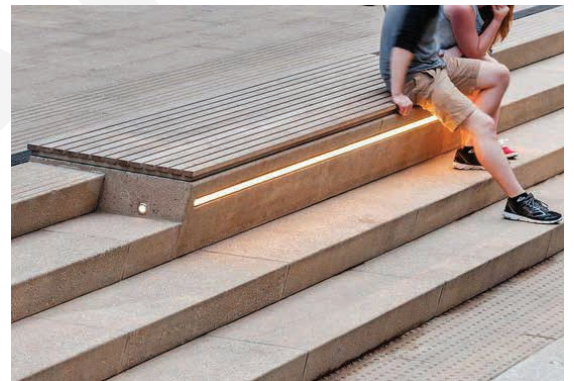
Precast concrete or natural stone seating steps
