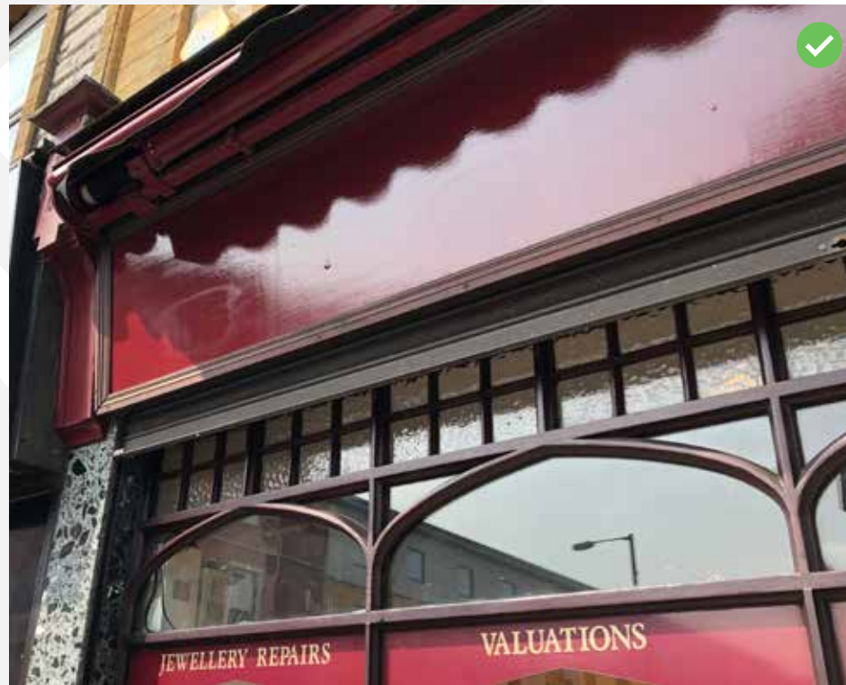
Figure 53. Well integrated, open type external shutter acceptable in necessary situations
