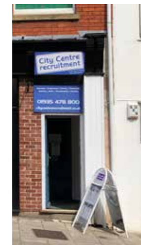
Figure 28. Signage disregards building elements
