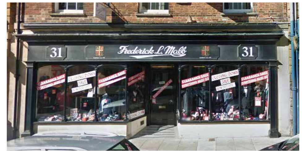
Figure 57. A well maintained timber shopfront
