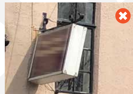
Figure 35. Bulky internally lit hanging sign detracts from building
